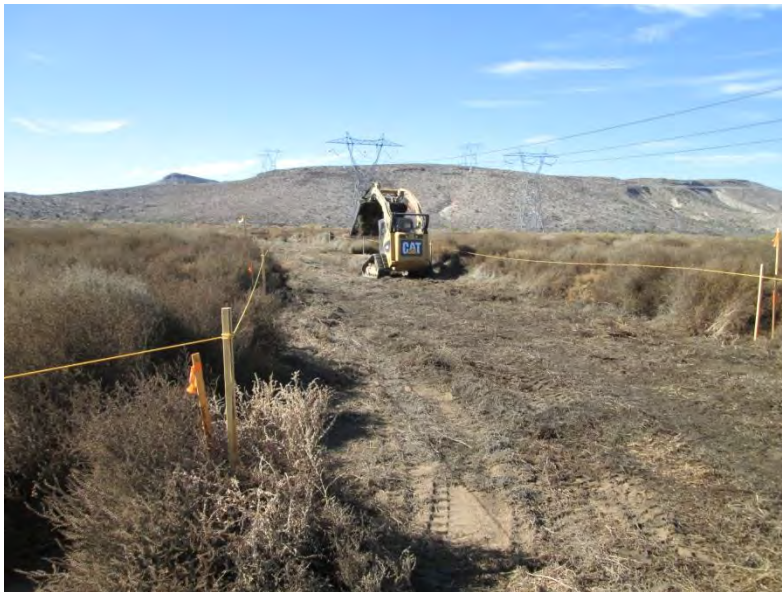
Photo 6: In accordance with MM-BIO-1a work activities associated with establishing access roads and pad sites for the 138 kV overhead construction component were observed being completed within the approved work limits. Staking and yellow rope is utilized to delineate the approved work limits.
